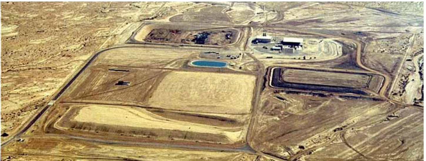
Aerial photo of hazardous waste disposal landfill facility in arid desert location. Final soil covers constructed with EMC SQUARED Stabilizer treatments approved by CalEPA for ongoing permanent closures as disposal cells are filled.
