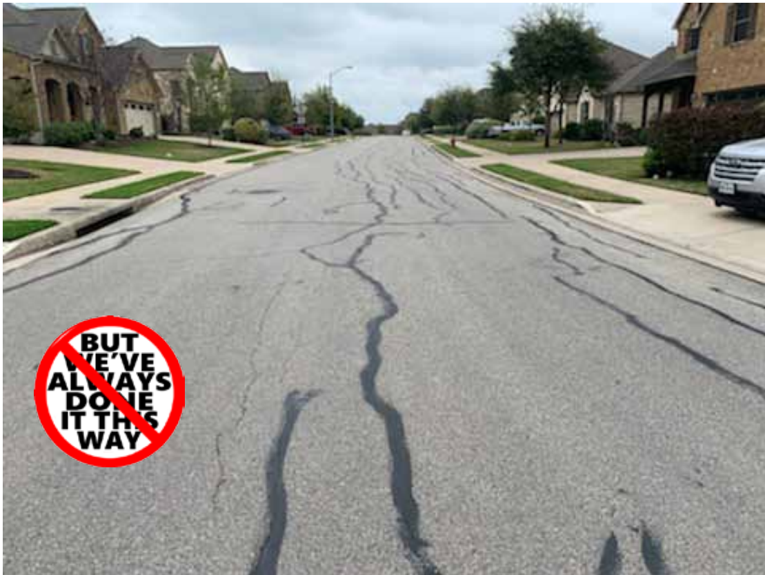
Teravista Community street subgrade soils treated with Lime
