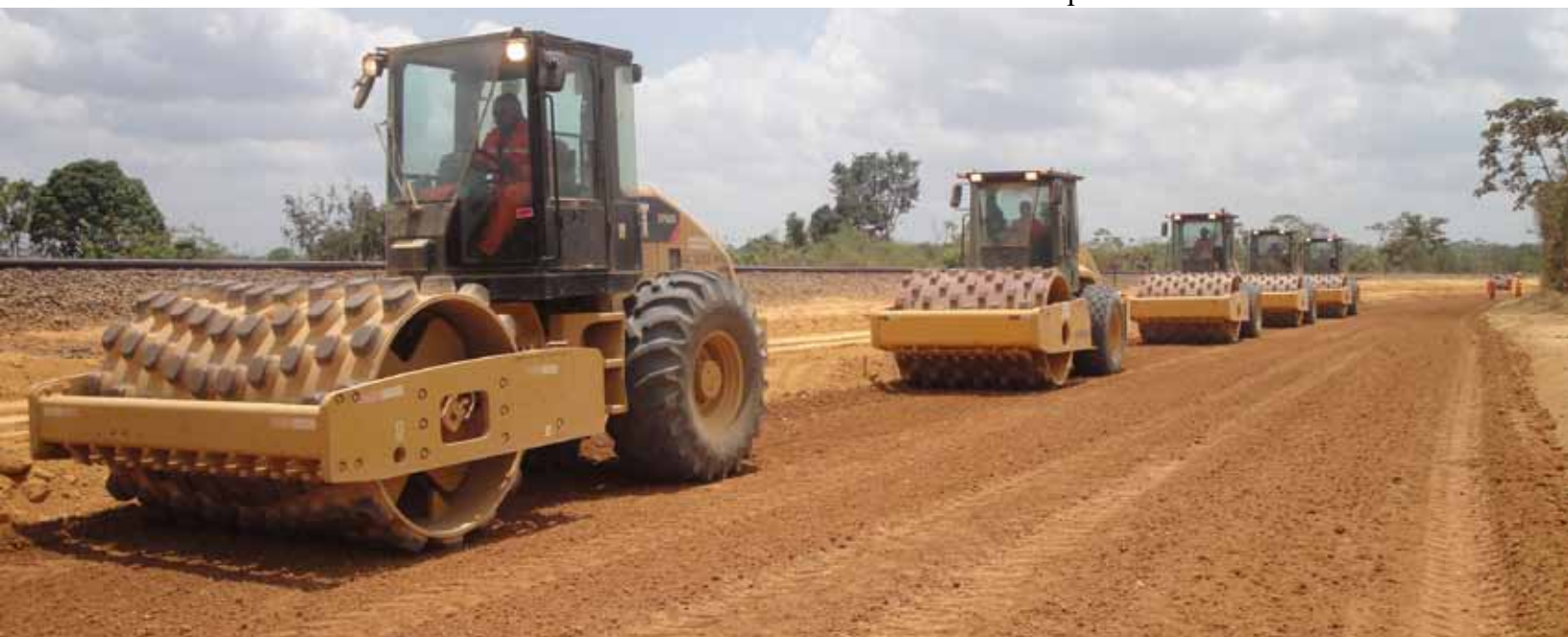
Compaction of EMC SQUARED System Stabilized Soils for New Railway
