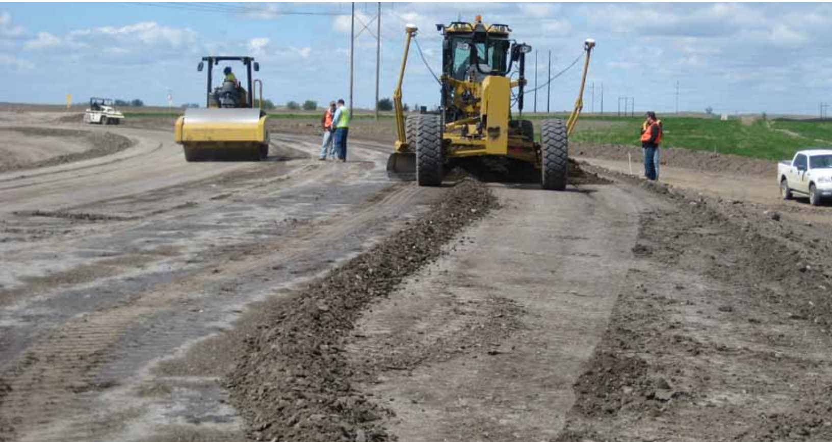
Road Project Under Construction Trimming and Final Compaction of Stabilized Subgrade
