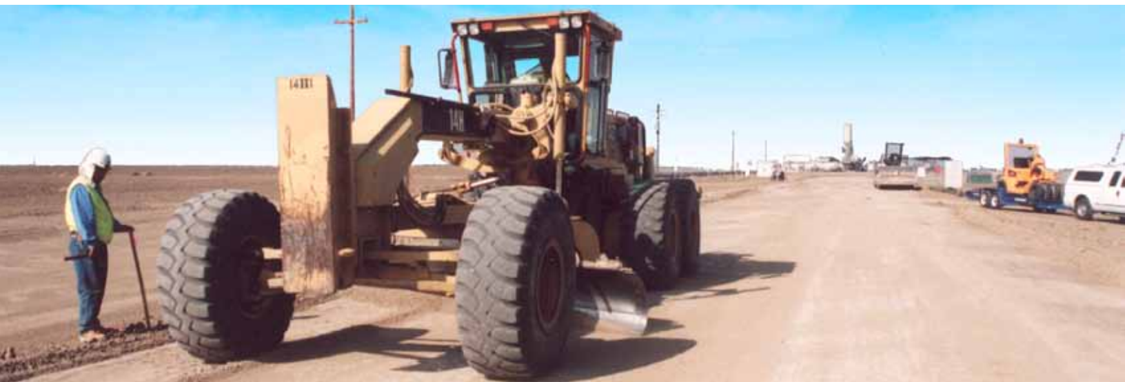
Road Project Under Construction Trimming and Final Compaction of Stabilized Subgrade
