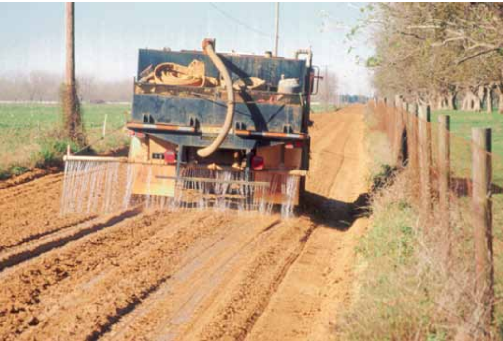
EMC SQUARED Liquid Stabilizer products being applied in Baldwin County, Alabama.
