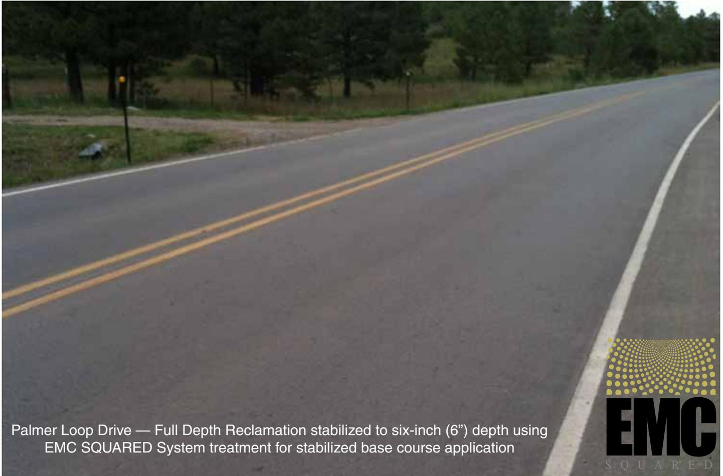
Palmer Loop Drive — Full Depth Reclamation stabilized to six-inch (6") depth using EMC SQUARED System treatment for stabilized base course application
