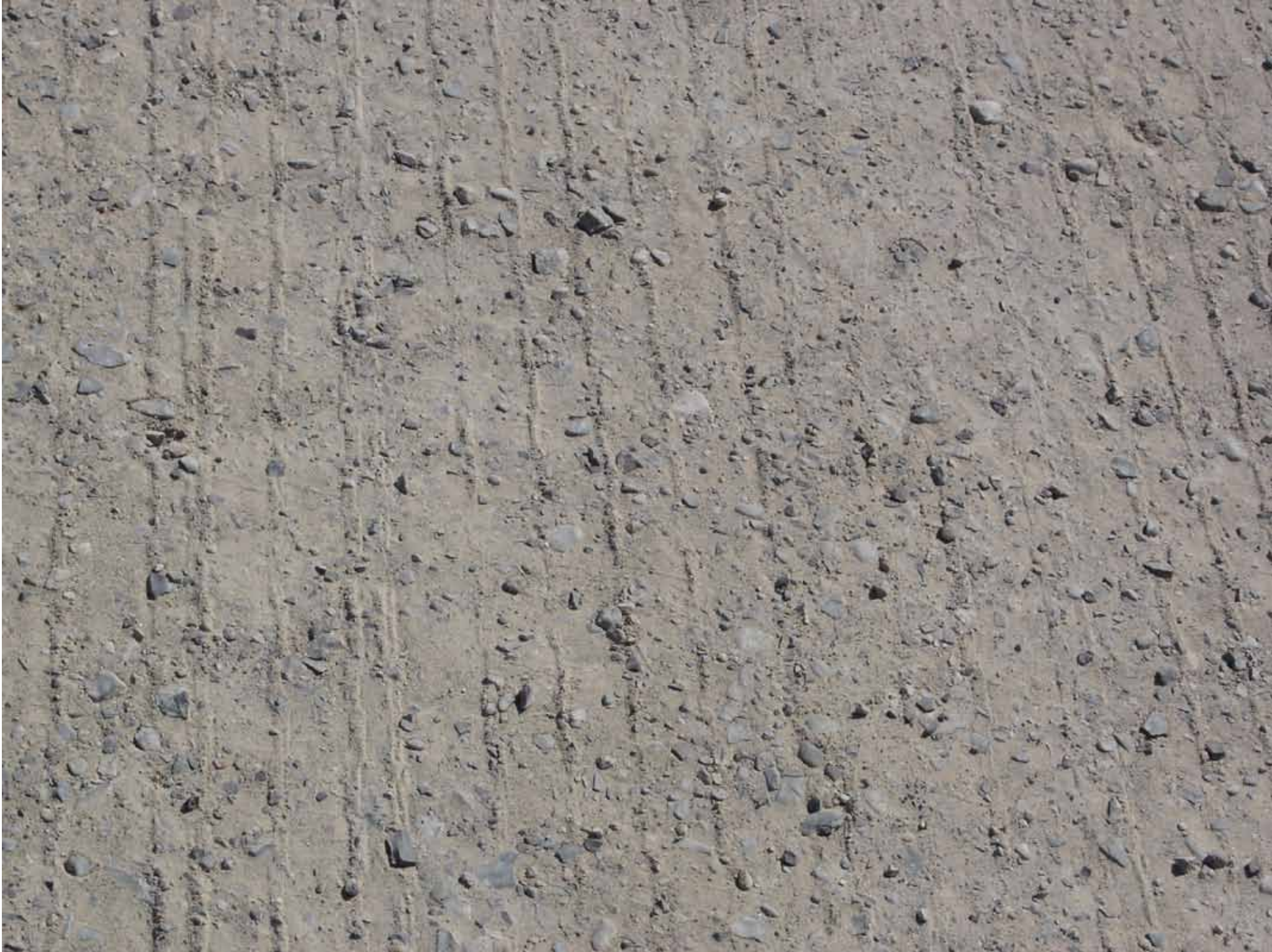
Close up of EMC SQUARED® Stabilized Aggregate road after passage of heavy haul truck
