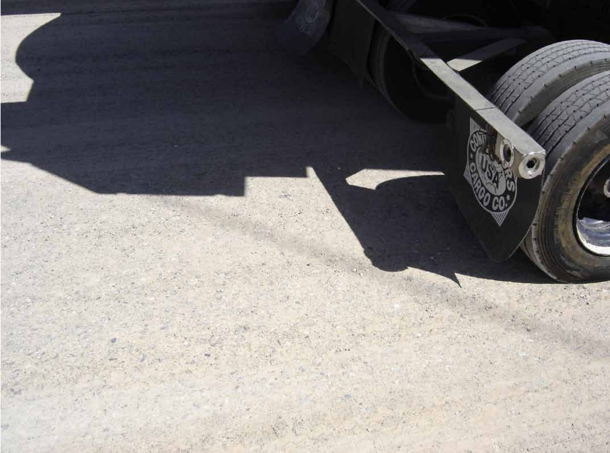
View of EMC SQUARED® Stabilized Aggregate road after passage of heavy truck.
