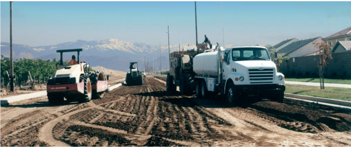
Compaction of stabilized subgrade soils with vibratory sheepfoot.
