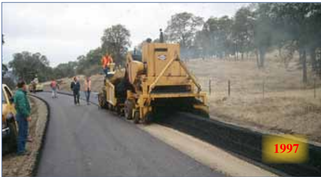
Placement of hot mix asphalt on stabilized, or "bound" base.
