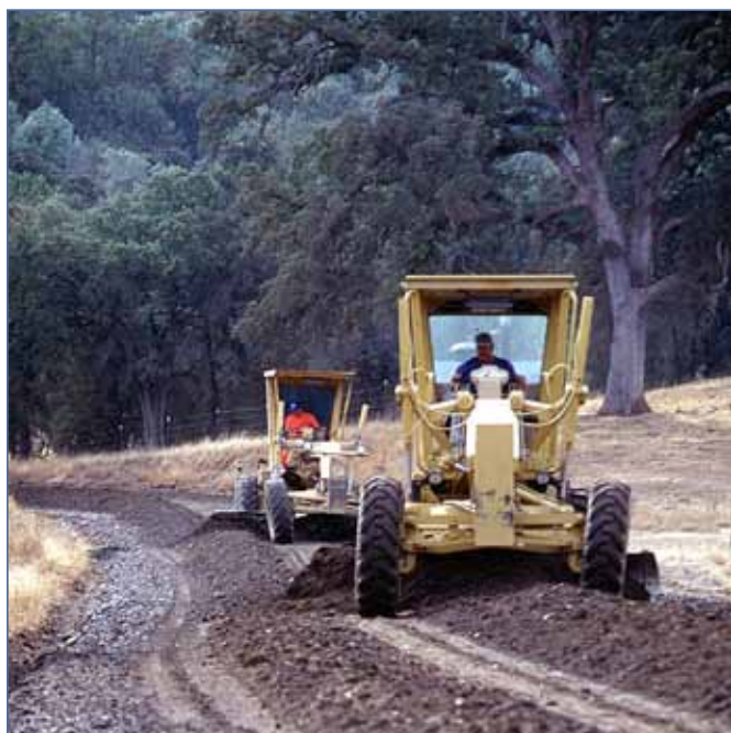
Following application of the liquid EMC SQUARED Stabilizer treatment to the asphalt millings and aggregate material, the treated aggregate mixture was processed by a tractor-drawn agricultural disk and motor graders, then shaped and compacted by vibratory smooth drum rollers.
