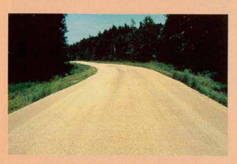
Photo shows the North West Angle Road in Minnesota. Even though the road is located in a wet, wooded area, use of liquid stabilizer reduced grading time and costs.
