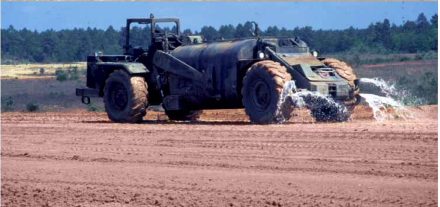
EMC SQUARED System stabilizer solution being applied to FLS clay capping soils by military water tanker.
