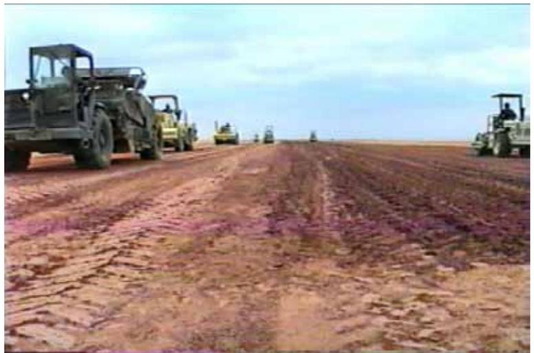
Water tanker applying stabilizer solution in front of cross-shaft rotary mixers with compaction equipment visible at right.
