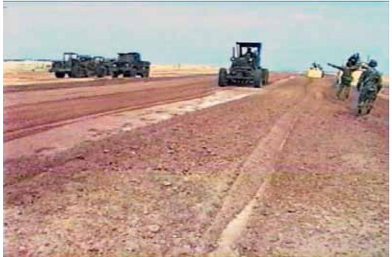
Water tanker application equipment parked at left while cross-shaft rotary mixer at distant right mixes stabilization treatment while soil and motor grader begins to grade and shape the treated soil.
