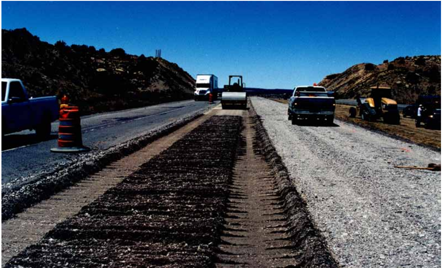
View behind Roto Trimmer showing compaction of the recycled pavement aggregate material in progress following pulverization and treatment with EMC SQUARED Stabilizer solution
