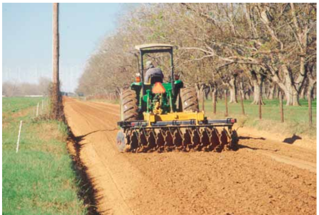
Stabilizer products being mixed into road soil before compaction in Baldwin County, Alabama.
