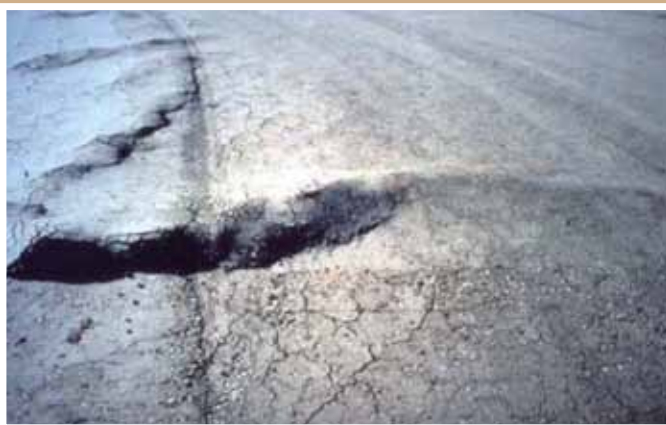
EXAMPLES OF SULFATE-INDUCED DAMAGE
