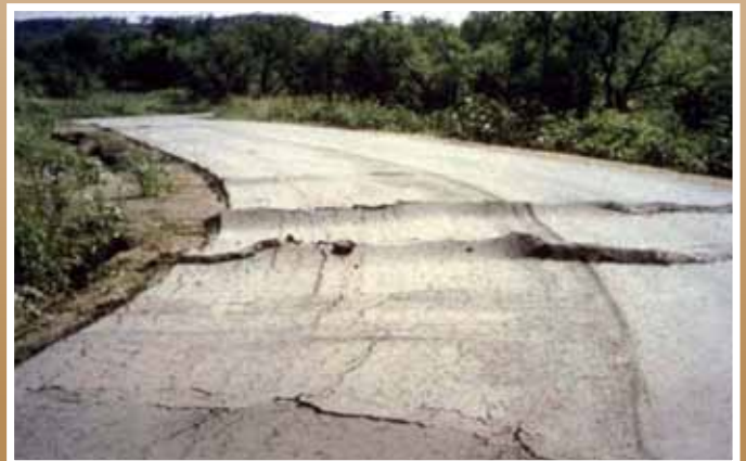
EXAMPLES OF SULFATE-INDUCED DAMAGE
