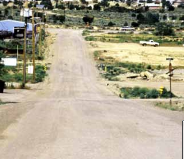
Aggregate Stabilized with EMC SQUARED® Stabilizer (utilized for two years as a street surface)
